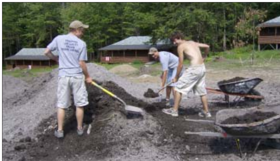
YCC crew spreading loam at Agassiz Village.
