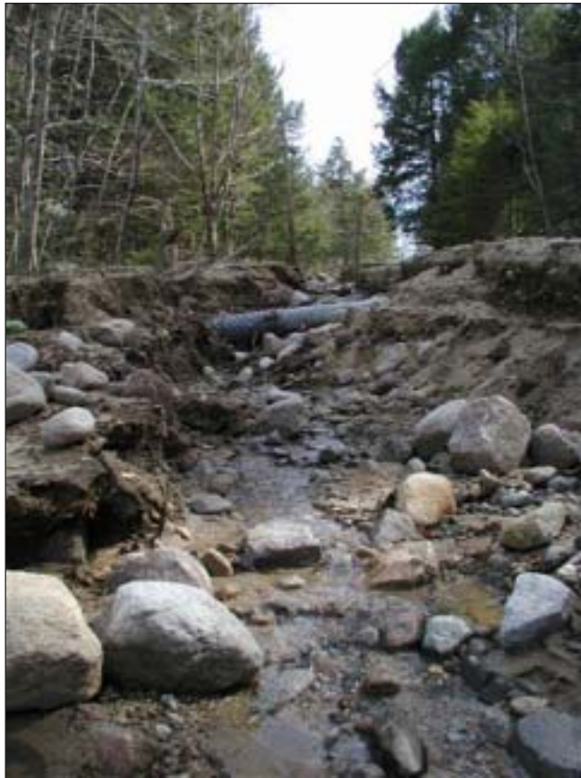
Patriot's Day Storm April 19, washes most of Otisfield's Parkway Road into Thompson Lake. (Photo Jane Fahey)
