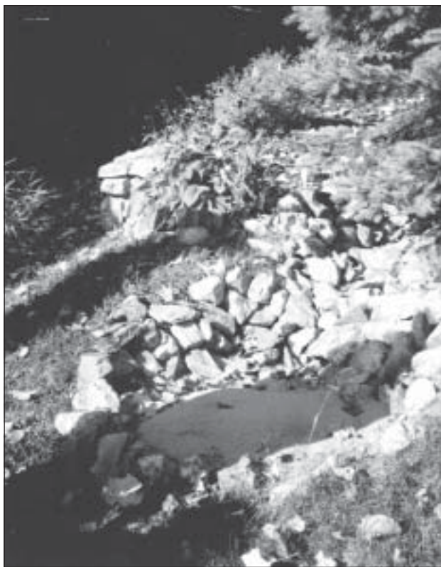
Settling pool on Canada Hill Shores Road installed by YCC.
